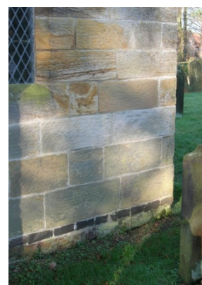
Fig 4 Exterior of vestry
