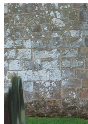
Fig 6 Exterior of north nave wall. Sealed Norman doorway
