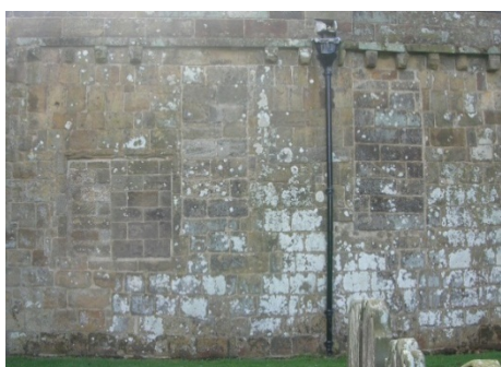
Fig 5 Exterior of north nave wall. Sealed window and doors
