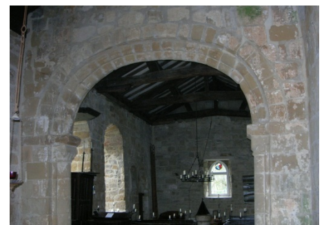
Fig 18 Chancel arch from the east
